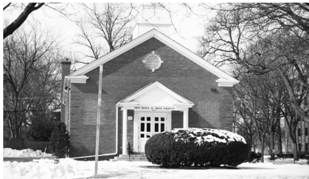
First Church of Christ - Small public/semi-public use along Harlem Avenue.
